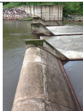
Ogee crest weir and stilling well
